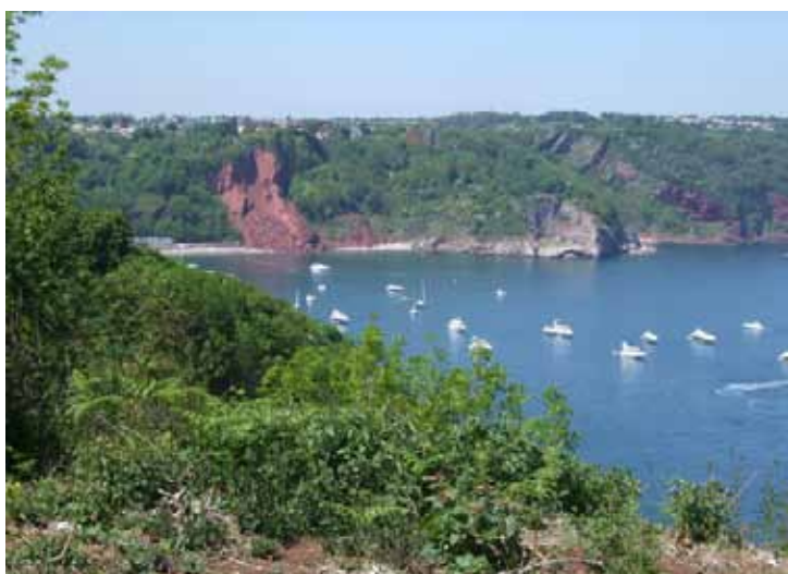
View across Babbacombe Bay to the cliff collapse at Oddicombe Beach
