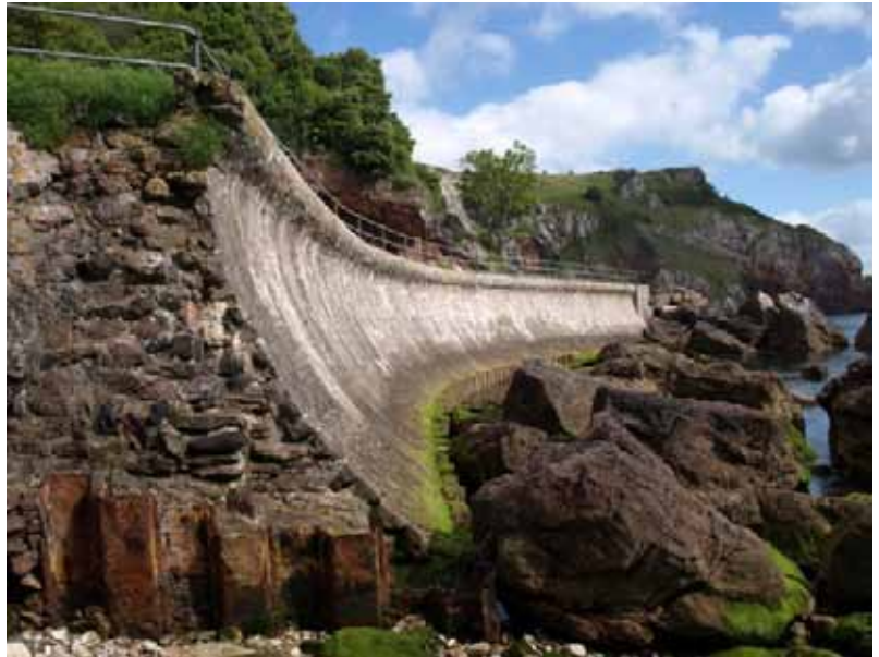
A concrete seawall protects Anstey's Cove from further undercutting © Derek Harper, Geograph (CCL)
